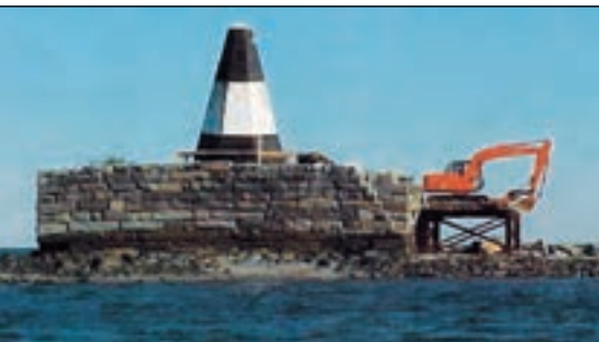
Atlantic Mechanical Inc. restoring Nixes Mate, 2003.
