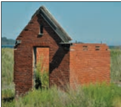
Remains of the Oil House.
